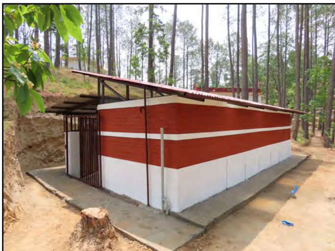
Completed sanitation block
